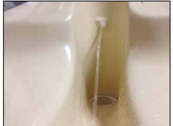
Connector Nozzle Draining into Base Where Waste/Water drains Into Waste Line (Over 4" Air Gap)
