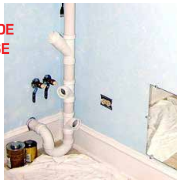
Waste Line coming Through "Head Wall"
