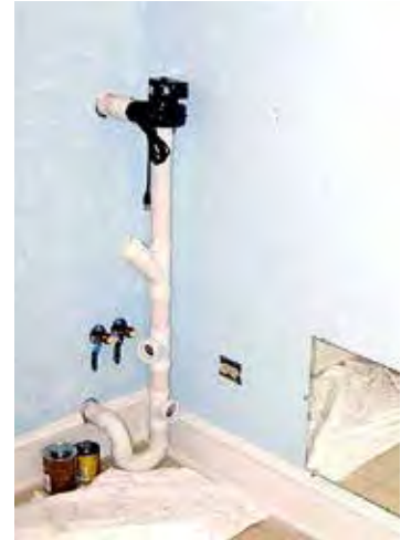
Option 2 Plumbing/Sewer Coming thru "Head Wall"
