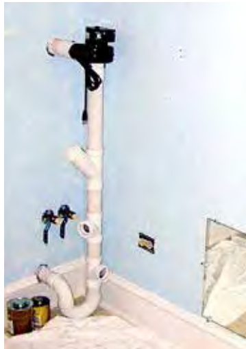
Sewer coming thru "Head Wall"
