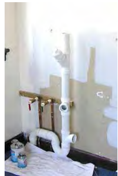
Option 3 Plumbing/Sewer Coming "Thru Floor"
