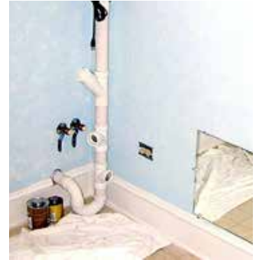
Option 2 Plumbing/Waste Line Coming through "Head Wall"
