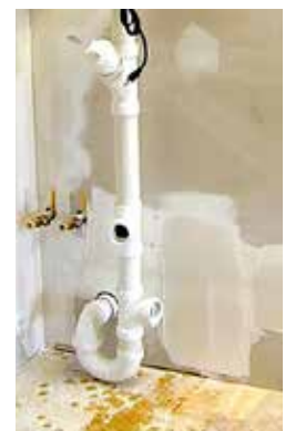
Waste Line coming Through "Cabinet Wall"
