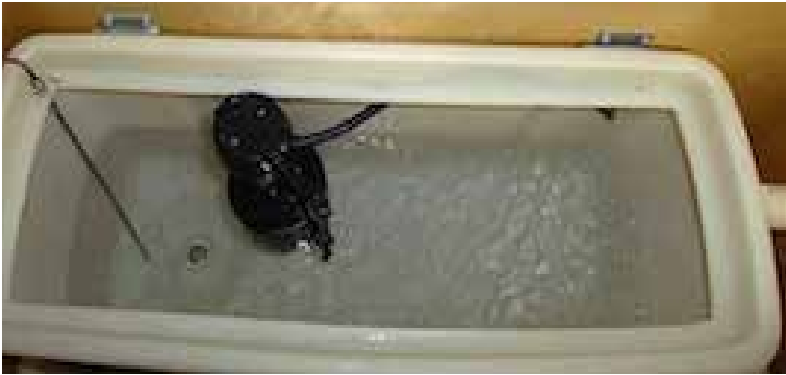
FLUIDMASTER 400 FILL FLOAT VALVE INSIDE WATER TANK (Anti Siphon Stands 1+” above the Overflow Inside Tank)
