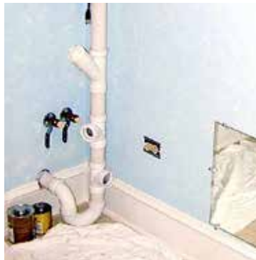
Waste Line coming Through "Head Wall"
